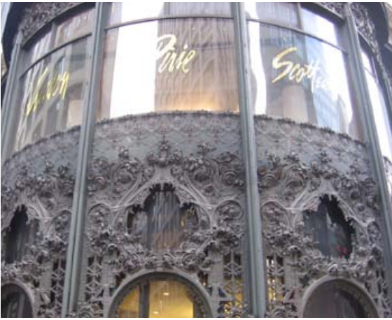
Target is expected to replace the century-old Carson Pirie Scott store in this Louis Sullivan-designed building in Chicago.
