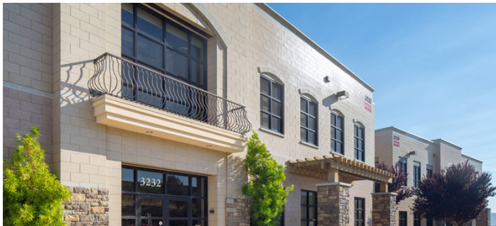
3196 CONSTITUTION DRIVE Formerly Livermore Charter School, now occupied by SMART Local Union,
